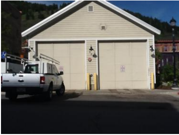
China Bridge Parking Garage Trash Compactor
